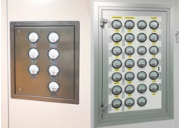
Stainless steel or HPL control board for rooms differential pressure gauge
