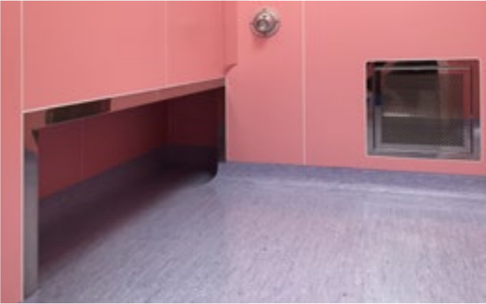
Air wall system and stainless steel flush perforated air return grilles
