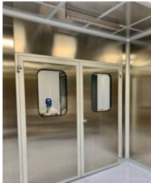
Stainless steel walls, doors and ceiling
