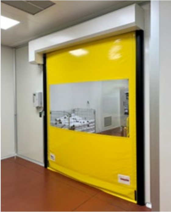
Roll-up door suitable for CNC or ISO 8 environments.
