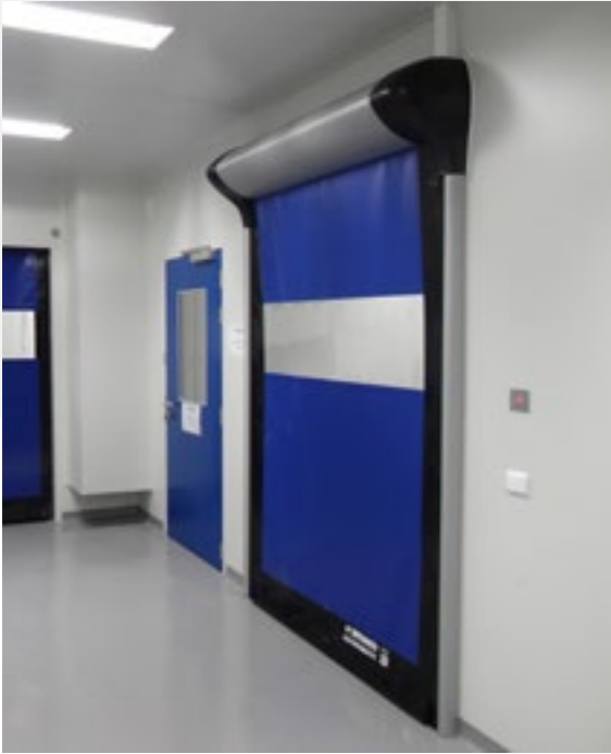
Air-tight roll-up door suitable for ISO 7 environments (in accordance to ISO 14644 -14)
