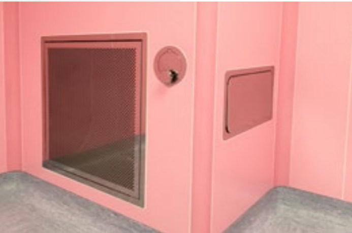
Air wall system and stainless steel flush perforated air return grilles
