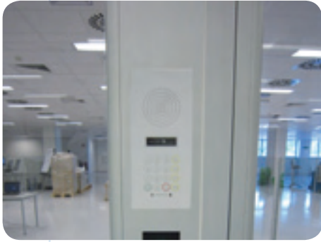
intercom in a technical panel
