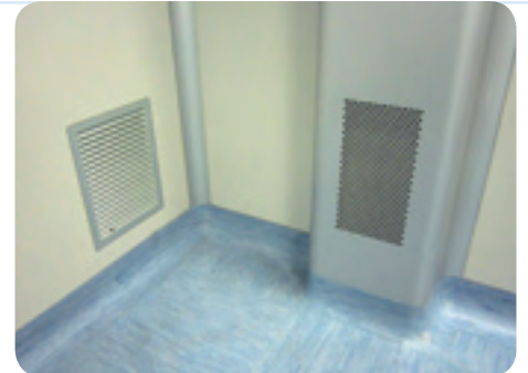
return air grills and Nicomac patent pending column
